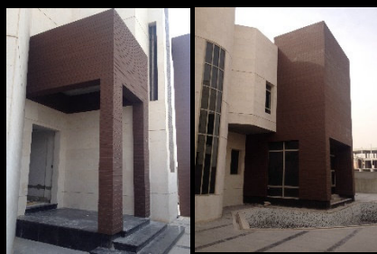
external wall cladding @ Qatar
